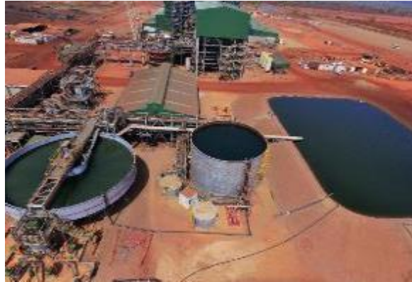
Process water storage
