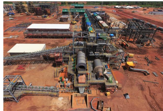
Ore bin (top) and primary mill and flotation (bottom)
