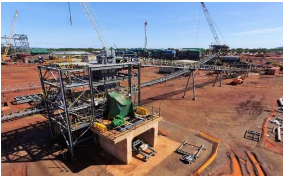
Figure 5 – Conveyor and recycle crusher system
