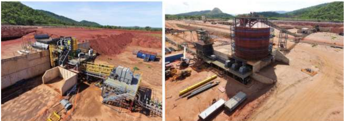
Figure 4 – Structural steel and mechanical equipment installation at the primary crusher (left) and installation of crushed ore bin storage, reclaim feeders and associated conveyors (right)
