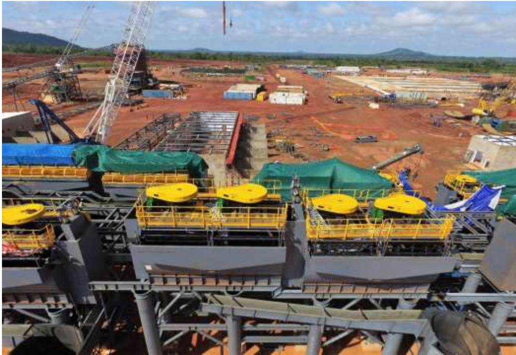
Figure 7 – All flotation cells have been installed
