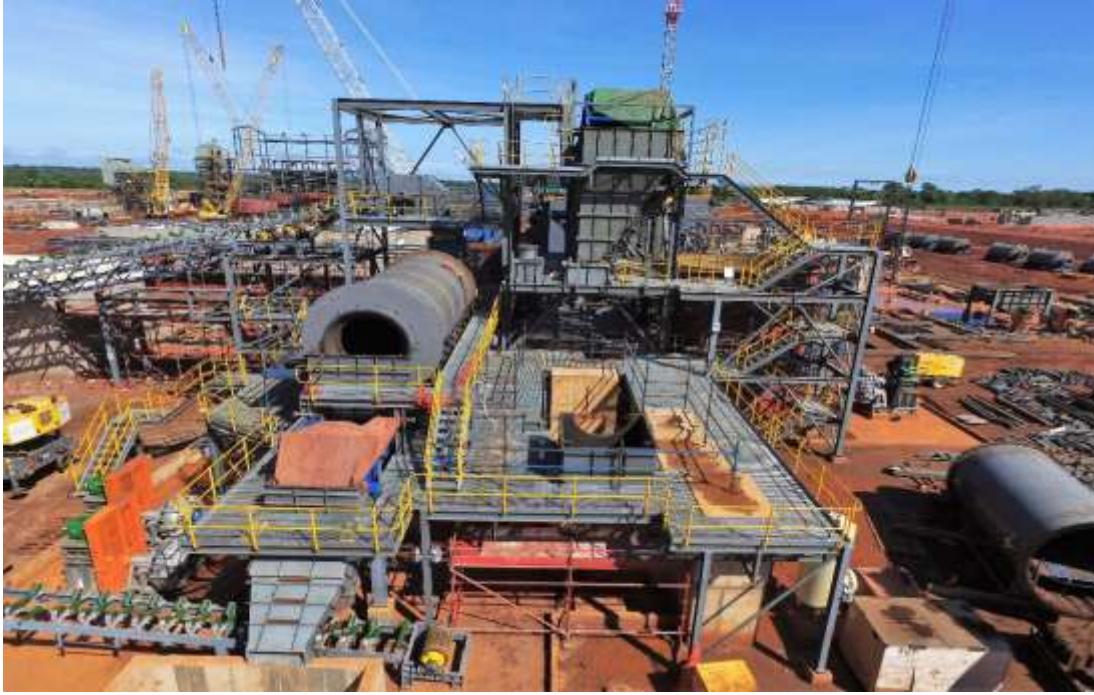
Figure 6 – Installation of scrubber and primary milling equipment prior to flotation circuit
