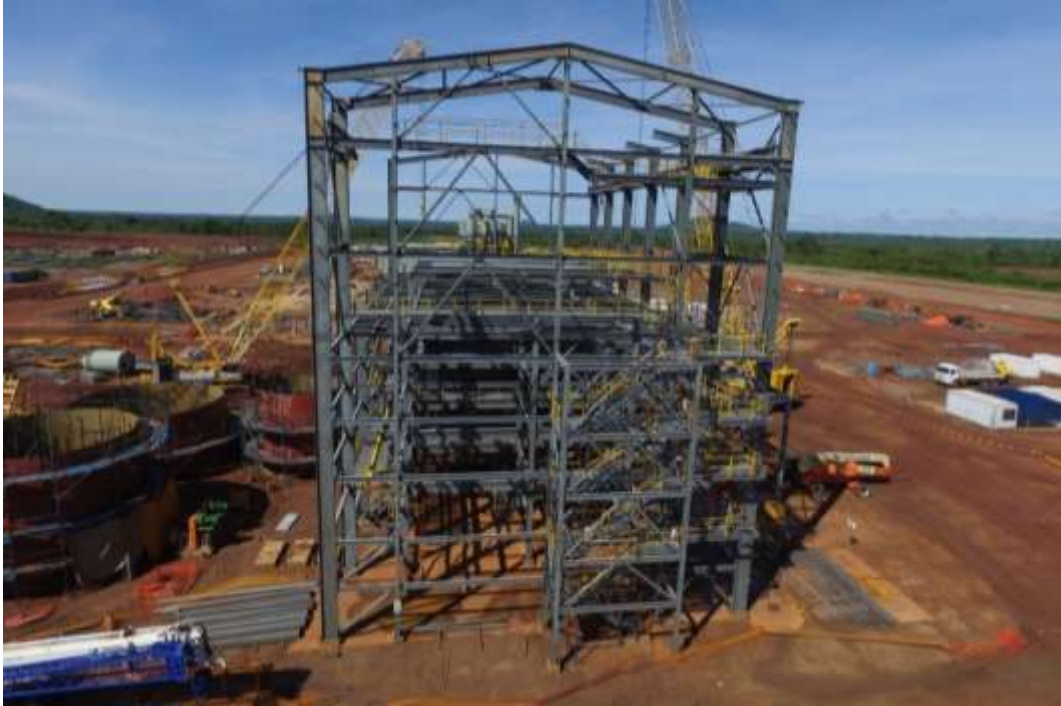
Figure 8 – Filtration building for dewatering graphite concentrate from the flotation area
