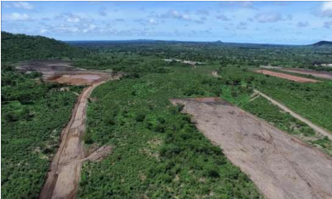
Figure 2 – Balama West haul roads, pre-stripping of Balama West pit, dumps and low grade stockpile
