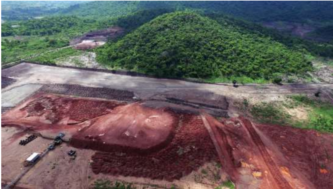
Figure 1 – ROM Pad Construction in Progress
