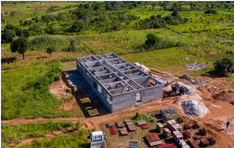
Balama Health Centre Upgrade (Surgery Block)
