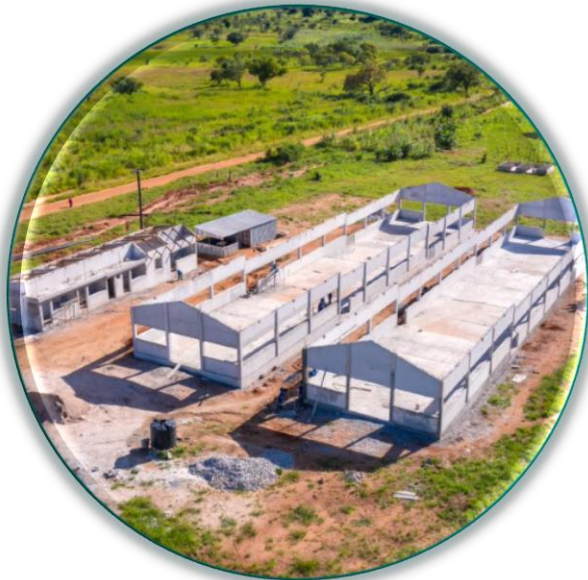
Construction of a central market in Balama
