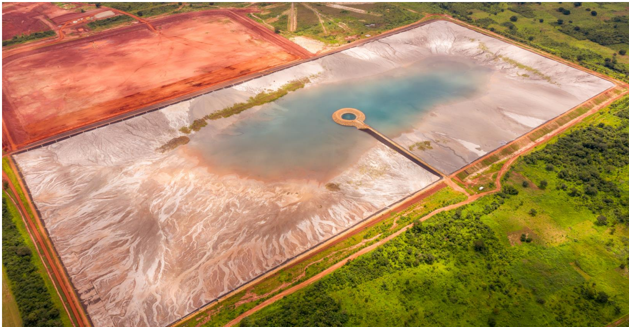
TSF cell 1 and TSF cell 2 construction
