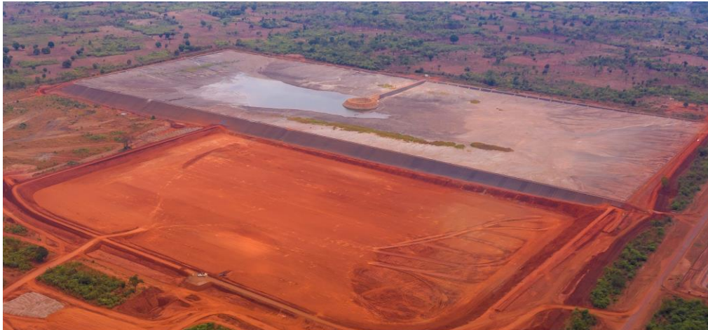
TSF cell 1 (top of photo) and TSF cell 2 construction
