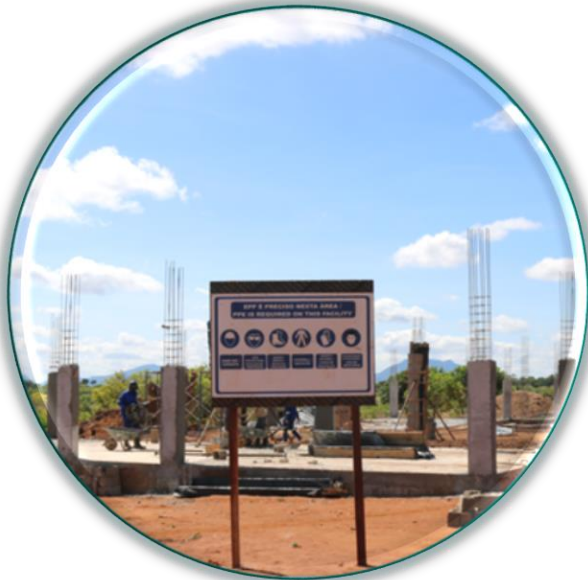
Construction of Balama Health Centre as part of the 2021-22 community projects
