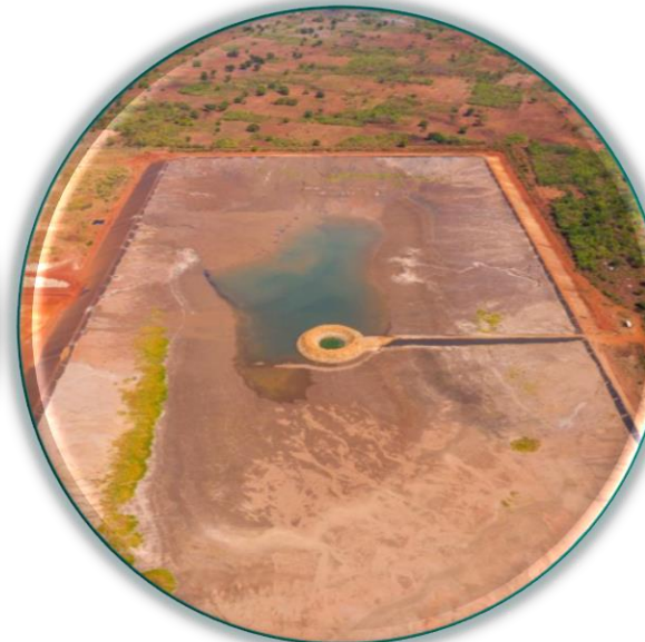
Balama Tailings Storage Facility Cell 1
