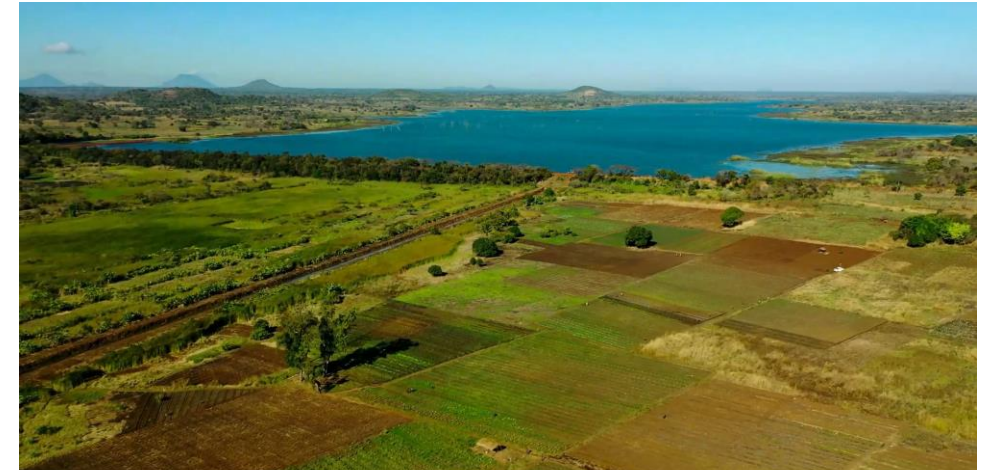
Aerial photo of Chipembe Dam and agricultural land partially supported by Syrah's Livelihood Development Program
