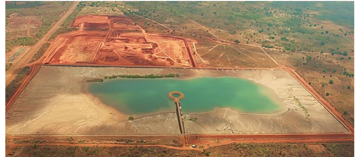
TSF Cell 2 Construction (top) and TSF Cell 1 (below)
