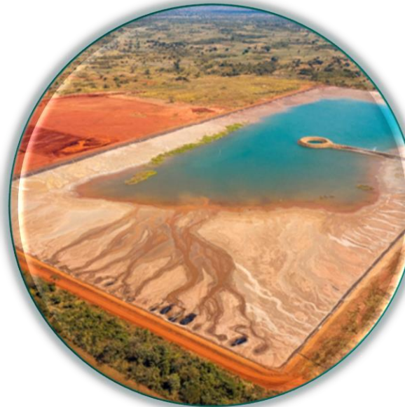
Balama Tailings Storage Facility Cell 1
