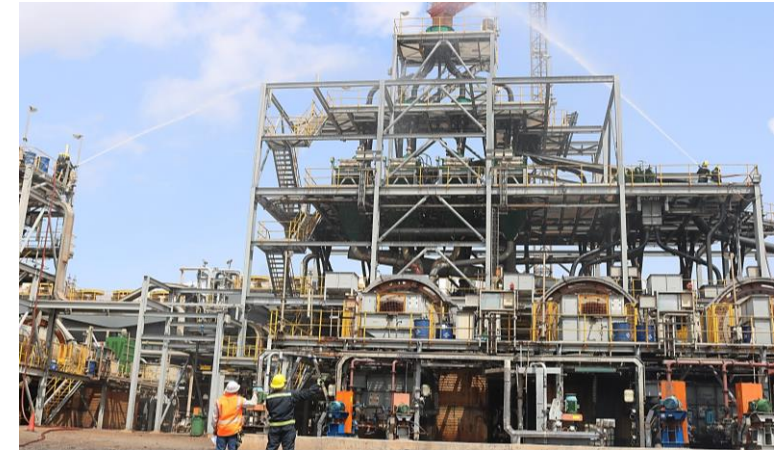
Employees engaged in firefighting training
