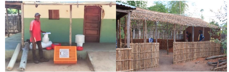
Poultry farmer in Ntete Village with new aivairy under construction
