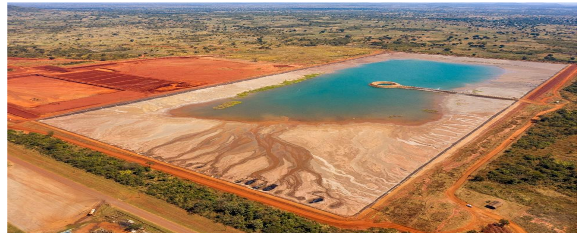
TSF Cell 2 Construction (left) and TSF Cell 1 (right)
