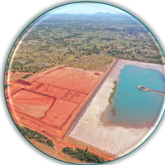
Tailings Storage Facility Cell 1 and Cell 2 (under construction)
