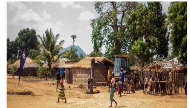
Rehabilitation of Maputo Road
