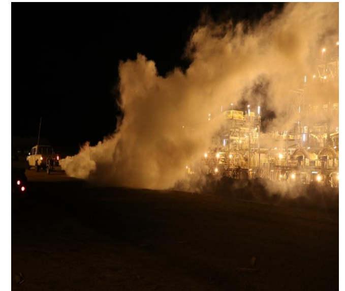
Mosquito fogging at the Plant Site
