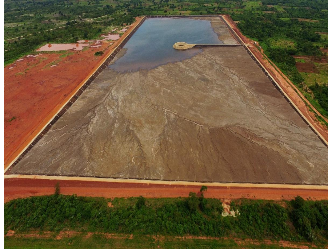
Balama Tailings Storage Facility
