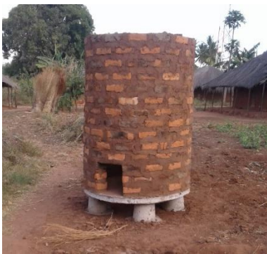
Grain storage unit construction
