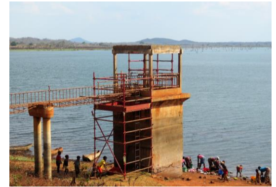
Dam valve access tower
