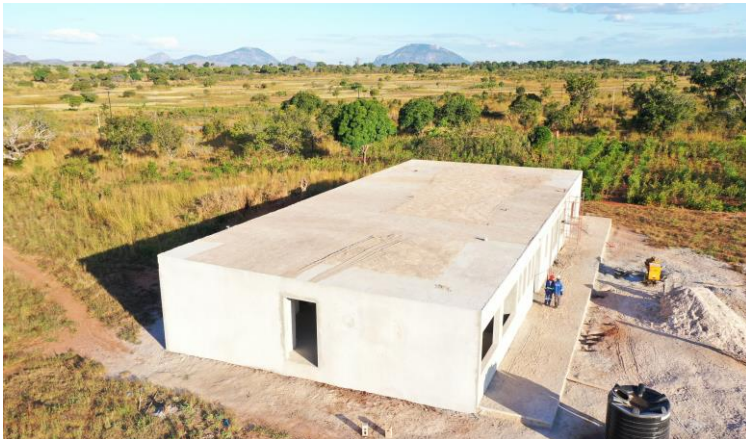
Balama Health Centre Upgrade (Surgery Block)
