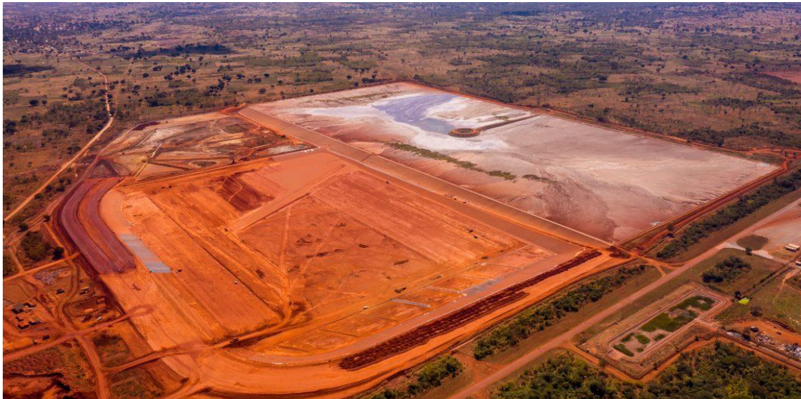
TSF Cell 1 (operational) and Cell 2 (under construction)
