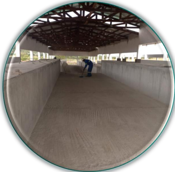
Construction of a central market in Balama
