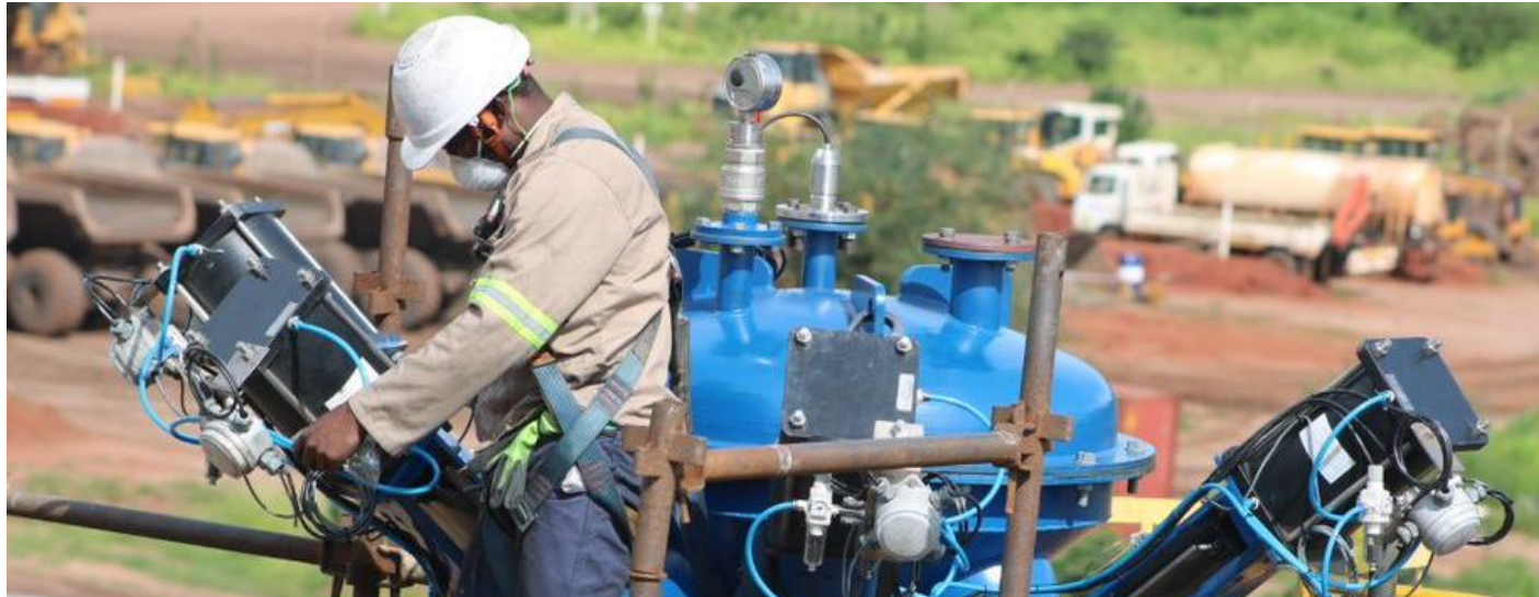
Balama maintenance employee adhering to the working at heights safety protocols
