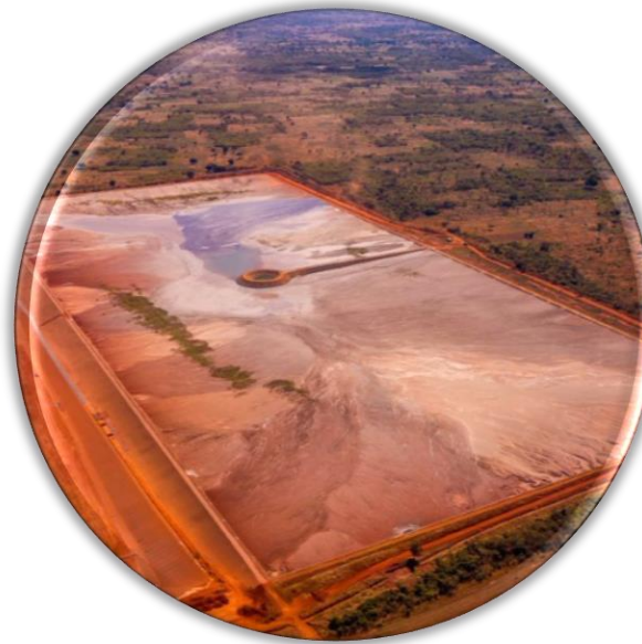
Balama Tailings Storage Facility
