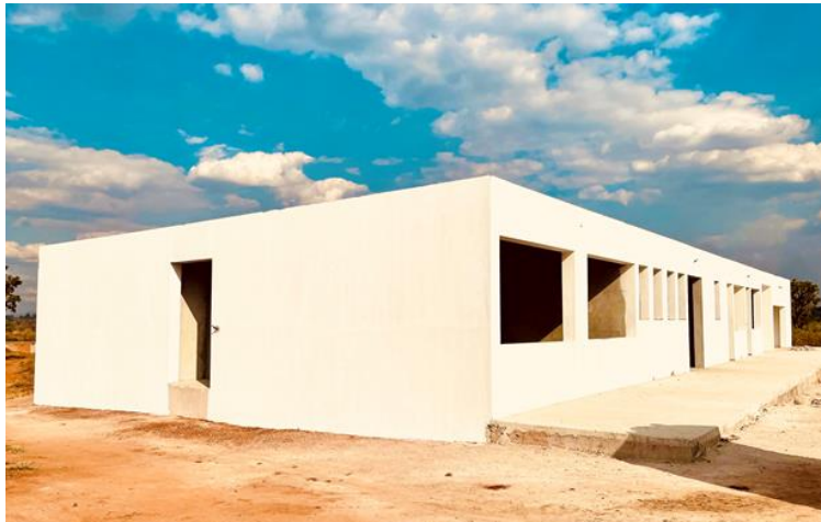
Balama Health Centre Upgrade (Surgery Block)
