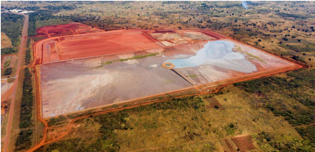
TSF Cell 1 (operational) and Cell 2 (under construction)
