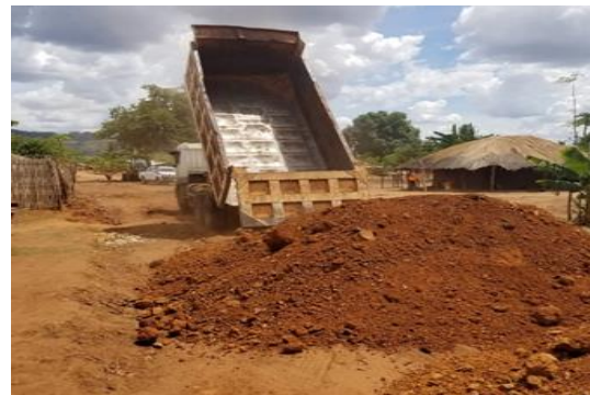
Rehabilitation of Maputo Road
