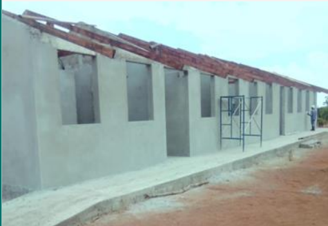
Primary school under construction in Muapé Village
