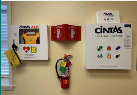
Ongoing focus on high risk assessments & safety training
