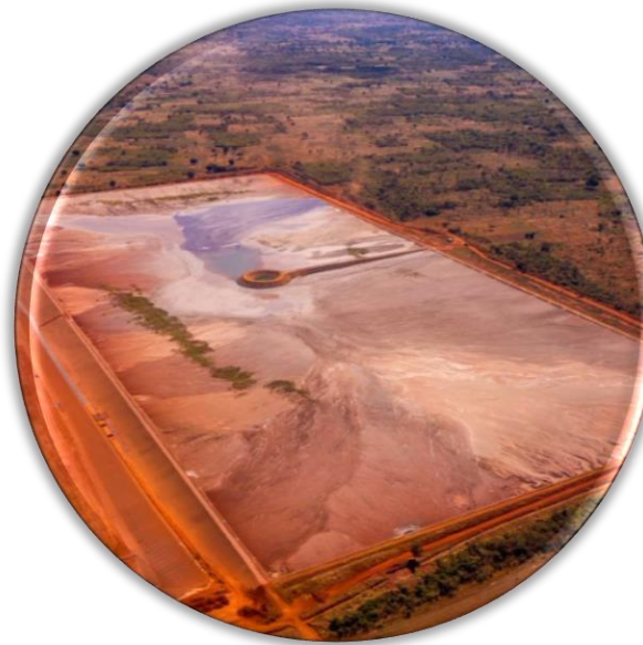
Balama Tailings Storage Facility
