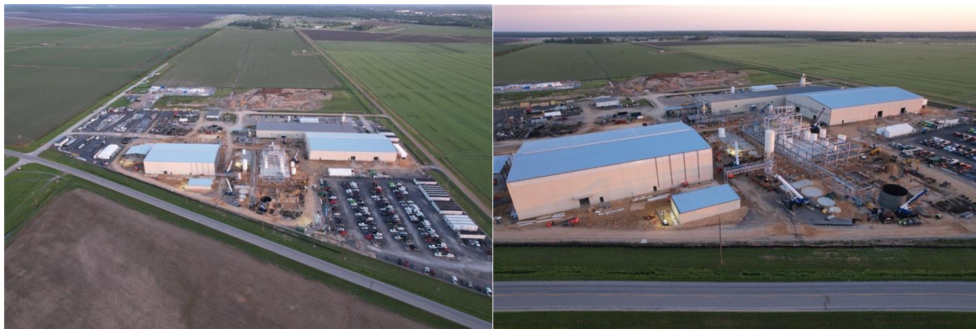
Figure 2: Construction of 11.25ktpa AAM Vidalia facility.
