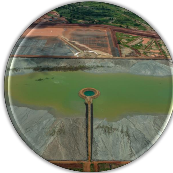
Balama Tailings Storage Facility monitoring
