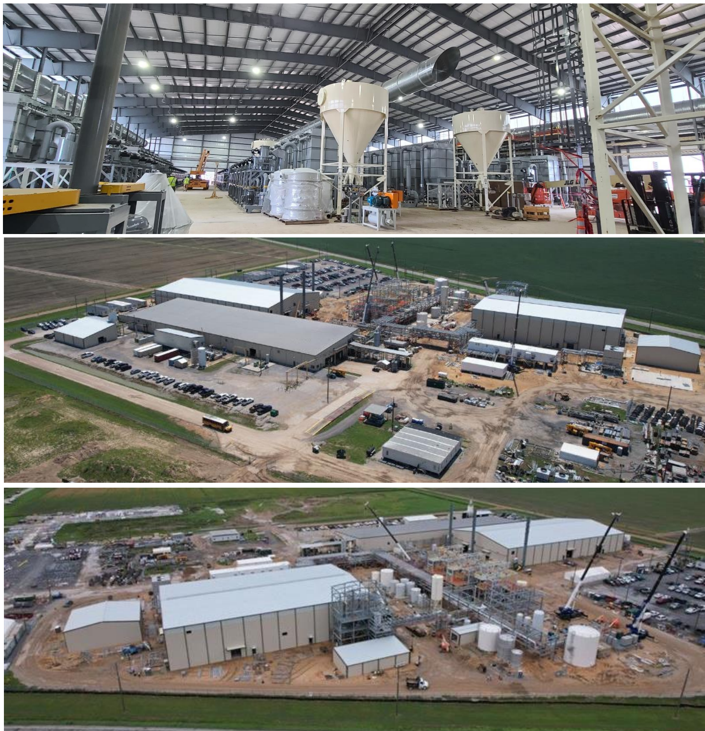
Figure 2: Construction of 11.25ktpa AAM Vidalia facility.
