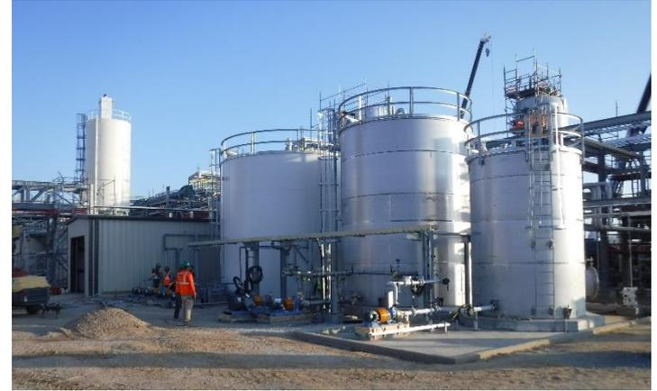
Figure 4: 11.25ktpa AAM Vidalia facility purification area (left); water and neutralisation discharge tanks (right).
