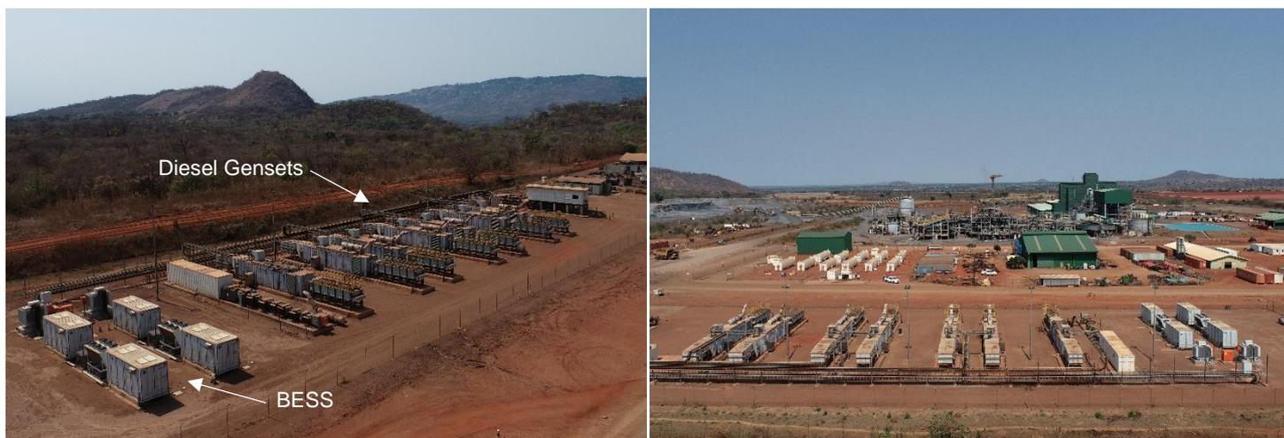
Figure 2: Balama BESS and Diesel Gensets.
