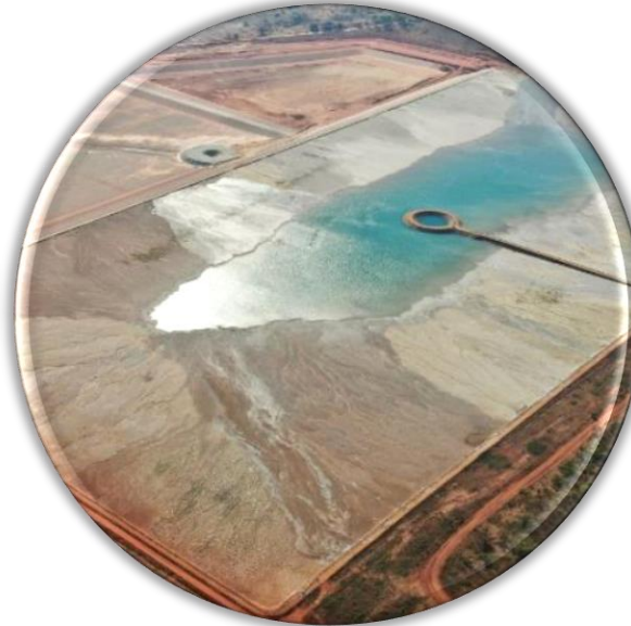
Balama Tailings Storage Facility monitoring
