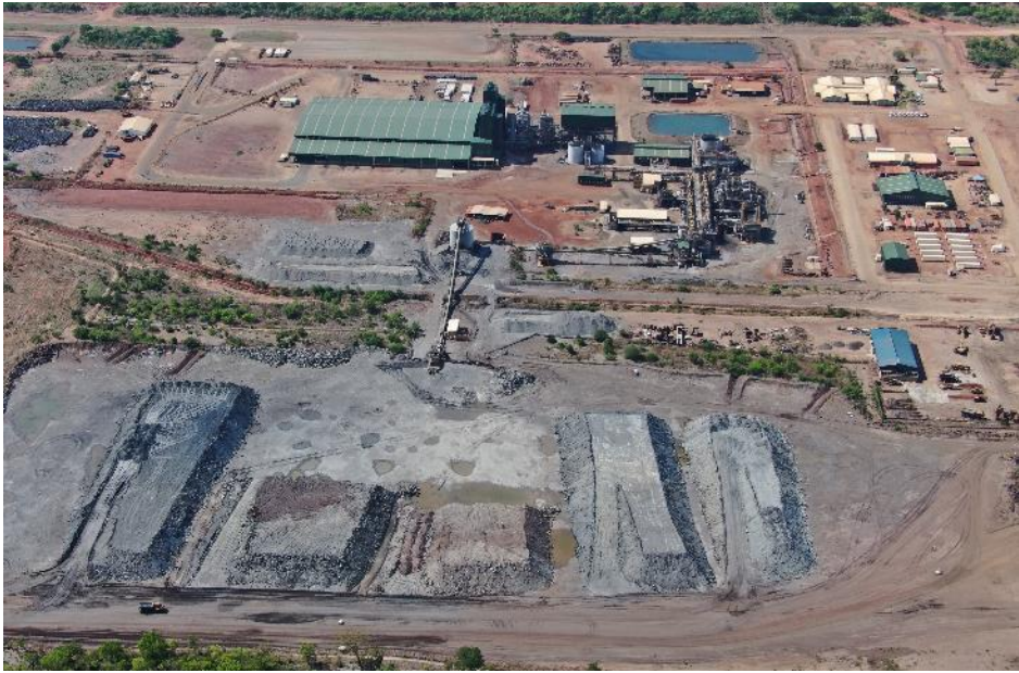
Process plant, product warehouse and ROM stockpiles
