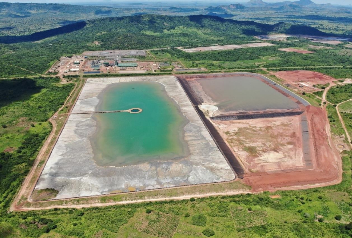
► Balama Tailings Storage Facility
