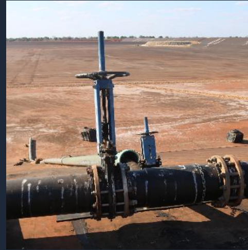
Balama TSF isolation valve and spigot
