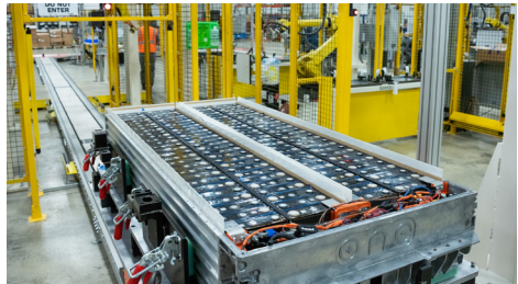
Aries LFP production line at Piston Automotive.
