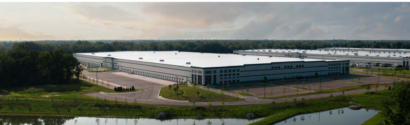
LFP cell and ESS module manufacturing at ONE Circle – Michigan, USA
