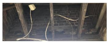
Near Miss 2 & 3 – workers were removing weatherboard cladding with crow bars when they discovered unknown old live electrical wiring beneath the surface
