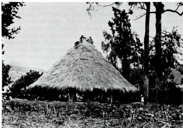
More than 400 Bahá'ís helped gather the materials for this meeting hut, built to house the Third Quechua Tantanakuy (All-Quechua Conference) in Otavalo, Ecuador. The building, a nine-sided affair of wood and thatched with straw, was 14 metres in diameter and sheltered over 450 Bahá'ís during the conference.
