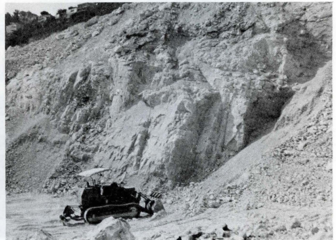
Excavating the site of the permanent seat of the Universal House of Justice: September 1975. An estimated period of five months will be required to remove more than 40,000 cubic meters of stone and earth. The completed excavation to an average depth of 10 meters (33 feet) will measure 150 meters by 250 meters (492 feet by 820 feet).
