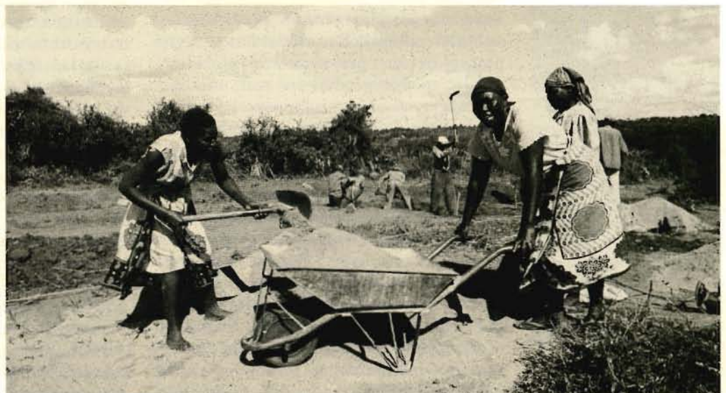
Members of the Kalimani Women's Group haul sand as part of a village water project that they are building. In the background, their menfolk dig the foundation for a water storage tank. The project will pull water from an underground reservoir created by a sub-surface dam on the nearby Mutendea River.
