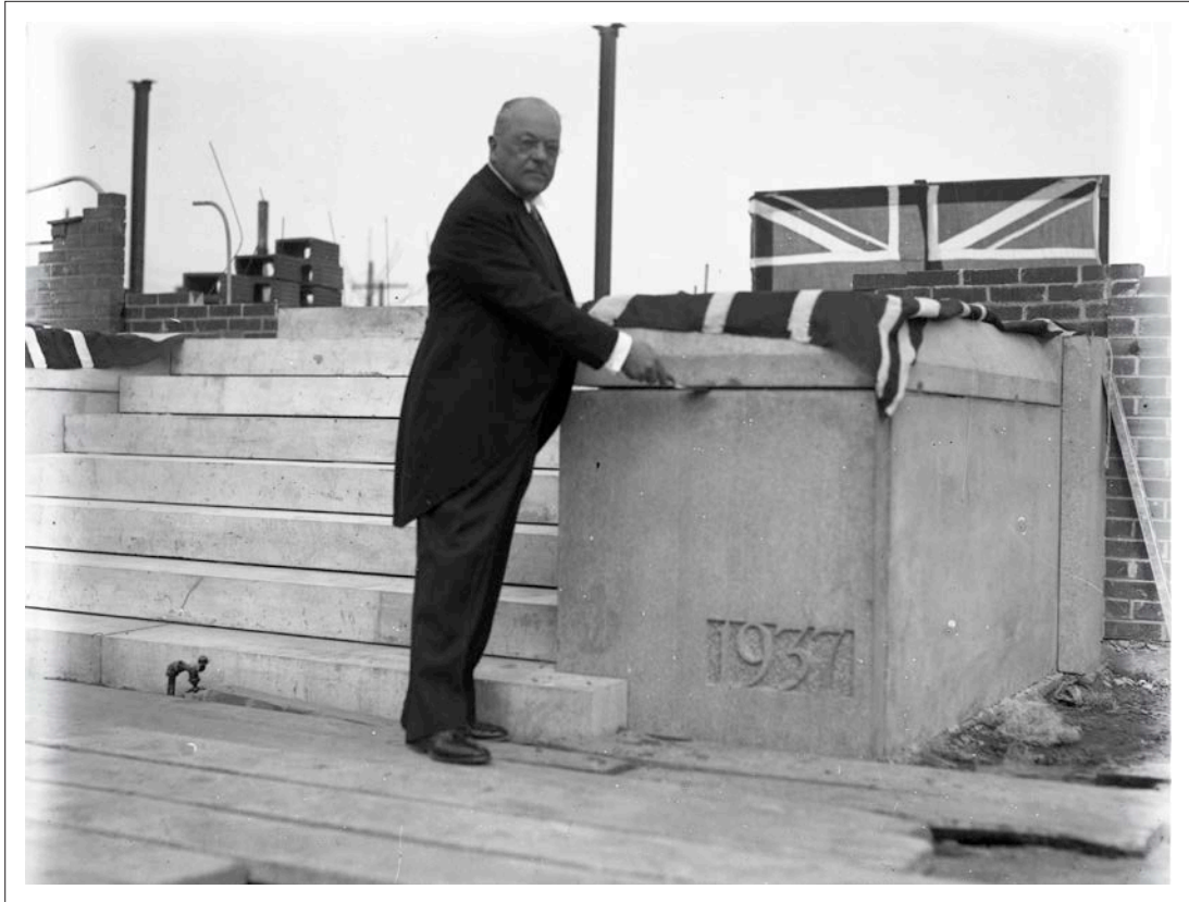
Gideon Sundback in 1937 laying the cornerstone at a building site for Lightning Fasteners in St. Catharines, Ontario, Canada. Courtesy of St. Catharines Museum, St. Catharines Standard Collection, S1937.17.2.1
