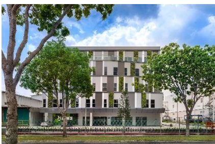
SOLAR REFLECTION Vertical fins on the facade screens solar heat from the Eastern Sun
