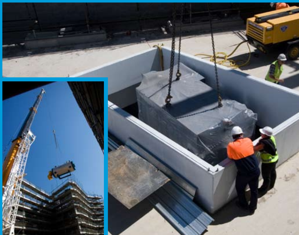
One of the trigeneration initiatives: Waste heat is captured by this Absorption Chiller (above) and uses it for heating in Winter and cooling in Summer.
