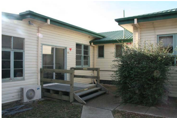
The external wall and roof cladding has been changed. Also note additional entrance (GBA, 2008)
