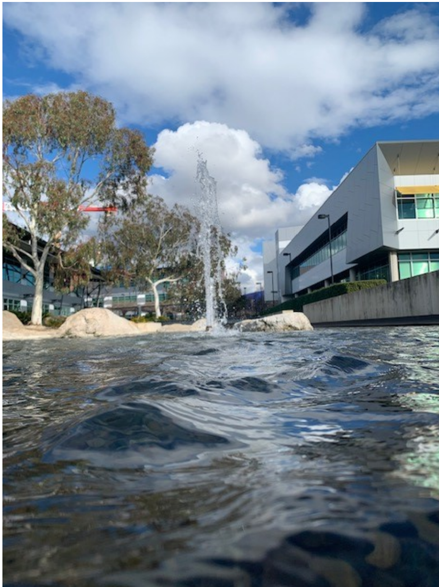
Stormwater Detention Basin at 2 Brindabella Circuit to settle and clean water through natural aeration
