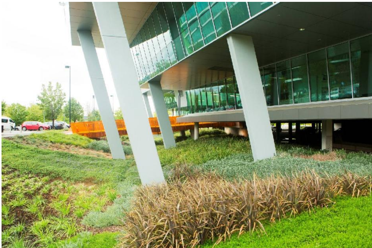
Figure 15.1 – landscaped swale, 3 Molonglo Drive, Brindabella Business Park
