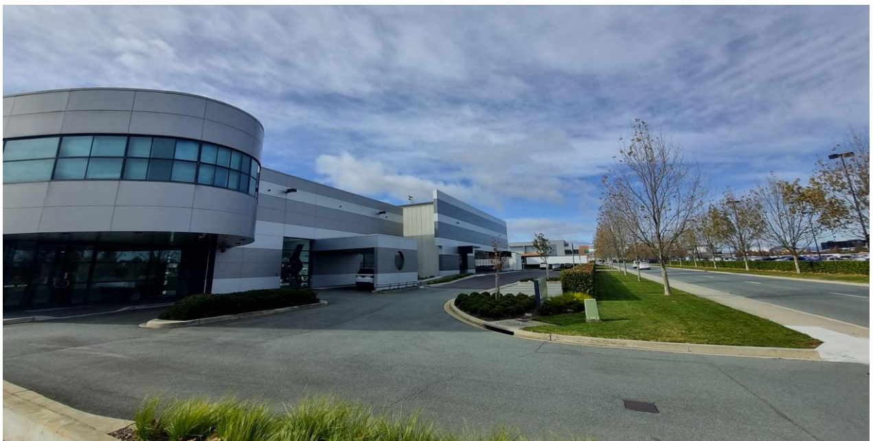
Capital Jet Hangar, George Tyson Drive Pialligo 2023
