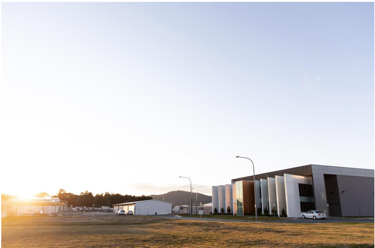
View of the recently (2022) demolished General Aviation Hangars (left), 14 Rayner Rd - (right) Pialligo, Canberra Airport
