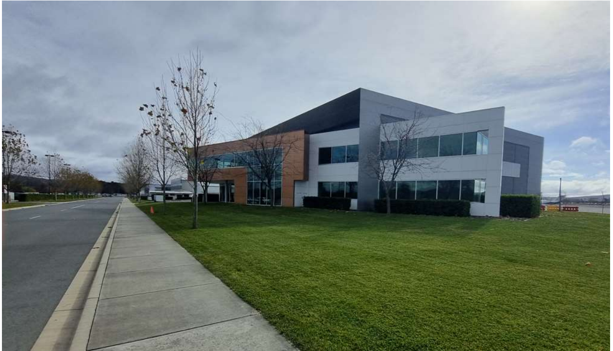
Office Spaces to a hangar, George Tyson Drive, Pialligo 2023
