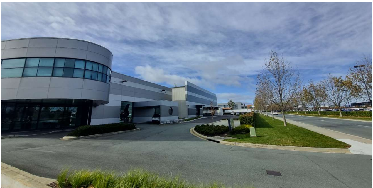
Capital Jet Hangar, George Tyson Drive Pialligo 2023
