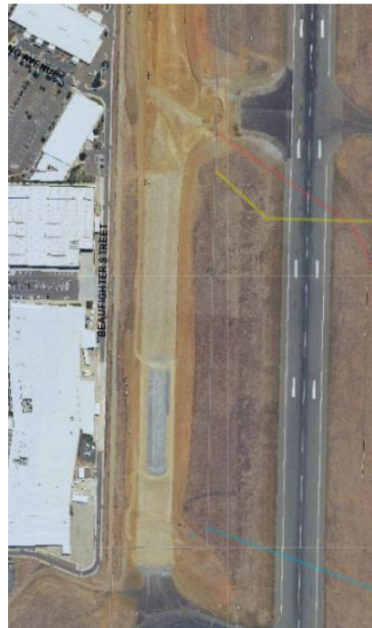
ACTMapi Image showing Taxiway Bravo under construction – January 2020
