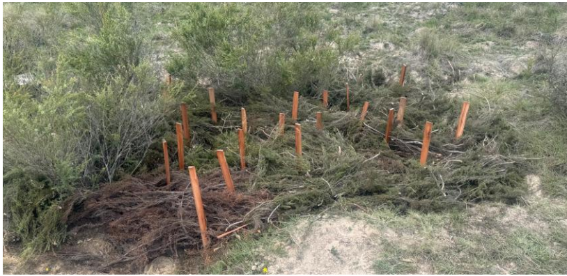
Using removed Kunzea parvifolia plants to stabilise areas of erosion/bare earth in ephemeral creek
