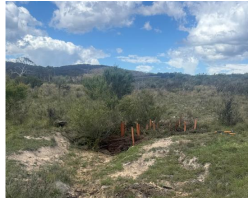
Using removed Kunzea parvifolia plants to stabilise areas of erosion/bare earth in ephemeral creek
