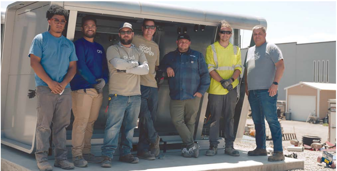
Torus Pulse™ installation at Schaeffer Metal Fabrication. Lindon, UT.
