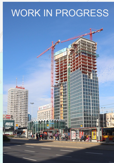
"Widok Towers, Warsaw under construction", Wistula, CC BY-SA 4.0, via Wikimedia Commons
