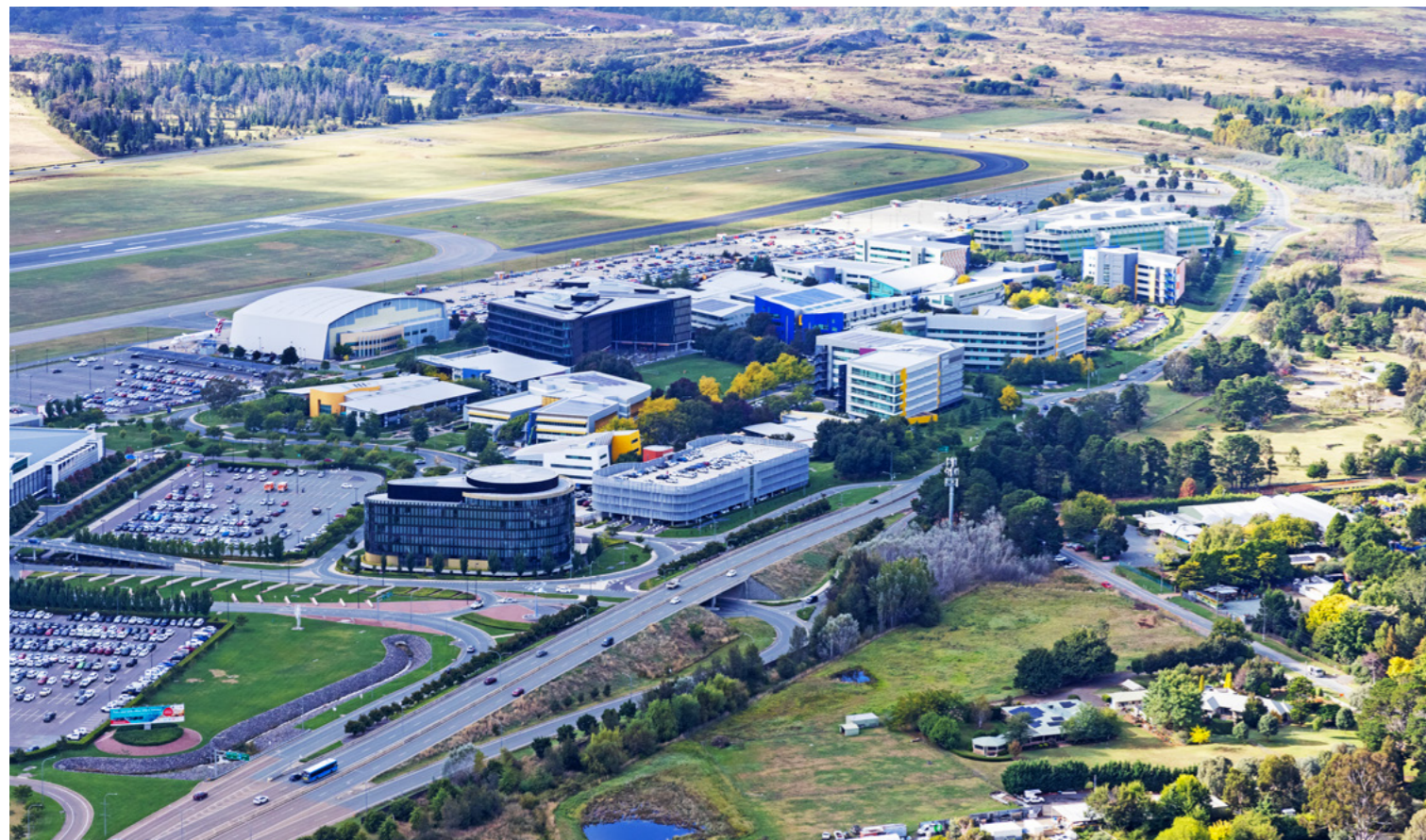
Located at Canberra Airport, Brindabella Business Park is an award-winning master-planned precinct consisting of 27 commercial office buildings.
