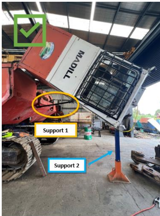
Hauler being worked on in the workshop. The cab maintenance/transport support is the primary support. Support 2 is the stand resting on the top of the cab.
