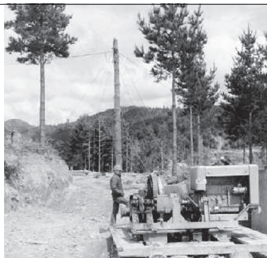
Stationary hauler with separate wooden spar
