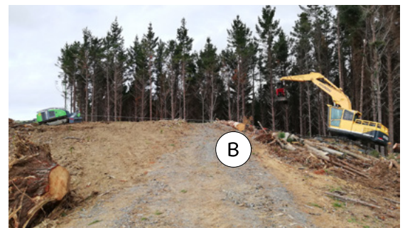
B Rub logs help keep the rope above dirt
