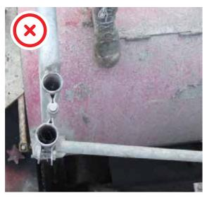
Exposed pipe ends create finger traps because the ends are not capped
