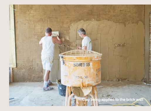
Clay, a natural product, has been applied as plaster on the walls. Clay has the lowest embodied  $CO_2$  of any interior finishes<sup>2</sup> as it does not demand any chemical treatments, and has a very low processing impact compared to traditional materials. It also helps ensure a better indoor climate in the shop.
